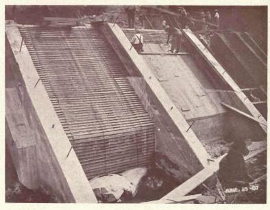
HOWING haunches on the up stream side of the buttresses. Notice in No. 2 the steel reinforcement being put in place and preparations being made for the placing of the deck slab, the varying thickness of which diminishing from the bottom to the top of the dam, is shown in the decreasing guage of the projecting rib.
